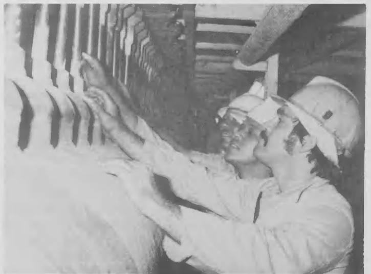
Two refinery units are undergoing major turnarounds. Above: the vacuum tower during the V3AR turnaround activities. Below: employees are inspecting the new pigtails at the H3AR unit.
